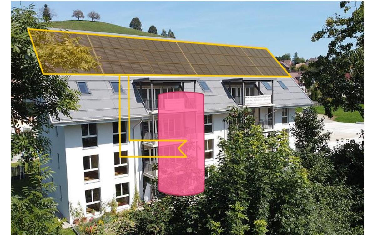
Conceptual illustration of the solar thermal system in the monitored MFH in Hütten
